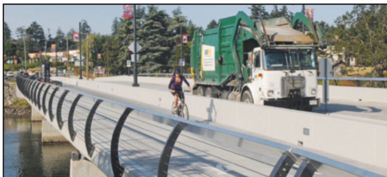
The new Craigflower Bridge in Victoria was built almost entirely with federal government money.
